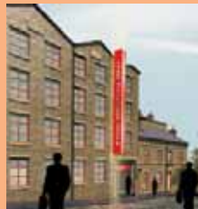
THE ELSIE WHITELEY MILL RE-USED
