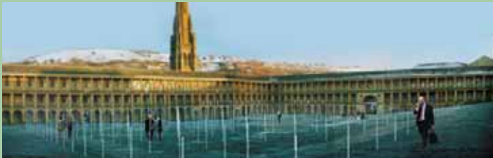
PIECE HALL COURTYARD FOUNTAIN
